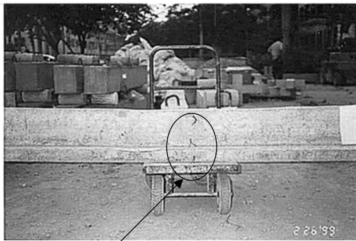
Fig.12 Failure on the bottom of Beam LRB
