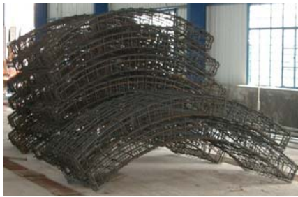
Fig.1 Segment reinforcement stacked on the ground
