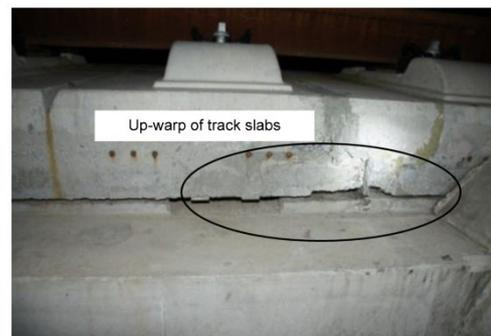
Fig. 3 Track slab up-warp on site
