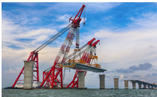
Fig. 6 Hoisting a span-scale girder segment using a floating crane
