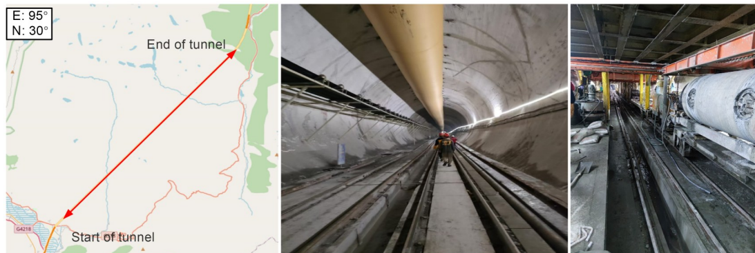
Fig. 1 Overview of the TBM tunnel project
