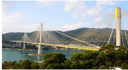
Ting Kau bridge
