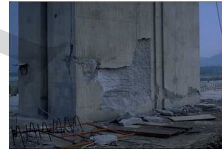
Stripping of Tower
