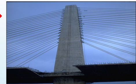
Rockfall of girder
