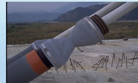
Retrench of cable
