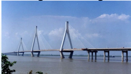
Dongting lake bridge
