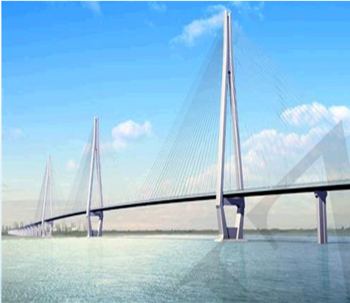
Prototype of a three-tower cable-stayed bridge
