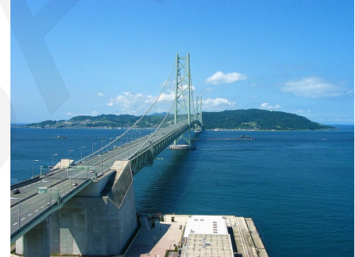
Long-span steel bridges
