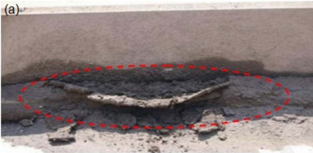
CAM damage (softening). Fig (a) Reprinted from (Zhu, 2014), Copyright 2014, with permission from Elsevier
