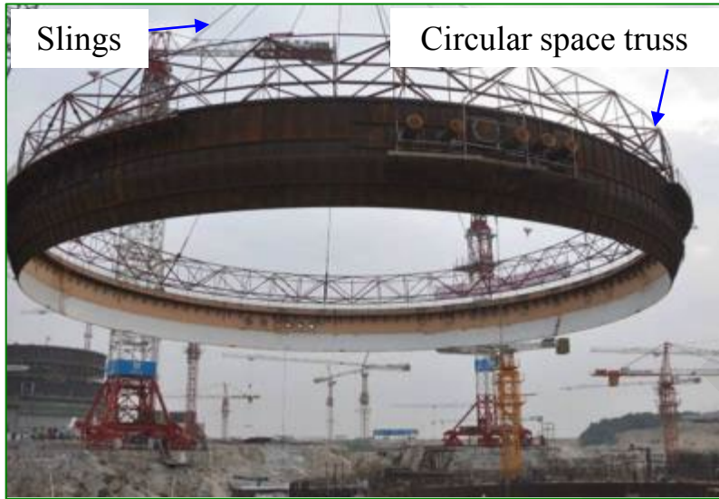
Lifting of the cylinder module
