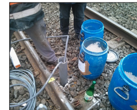
Installation of embedded accelerometers and geophones
