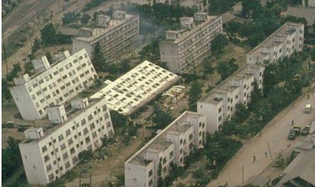
Loss of bearing capacity (1964 Niigata Earthquake)
