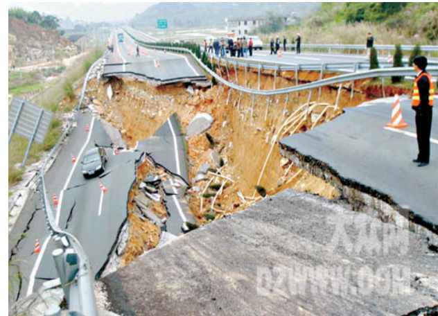
Failure of ground with columns
