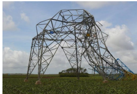
Out-of-plane buckling collapse of transmission tower
