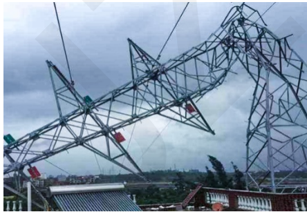
Out-of-plane buckling collapse of transmission tower
