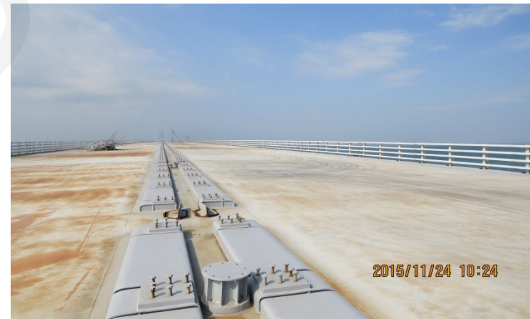
On-site picture after completion of steel box girders
