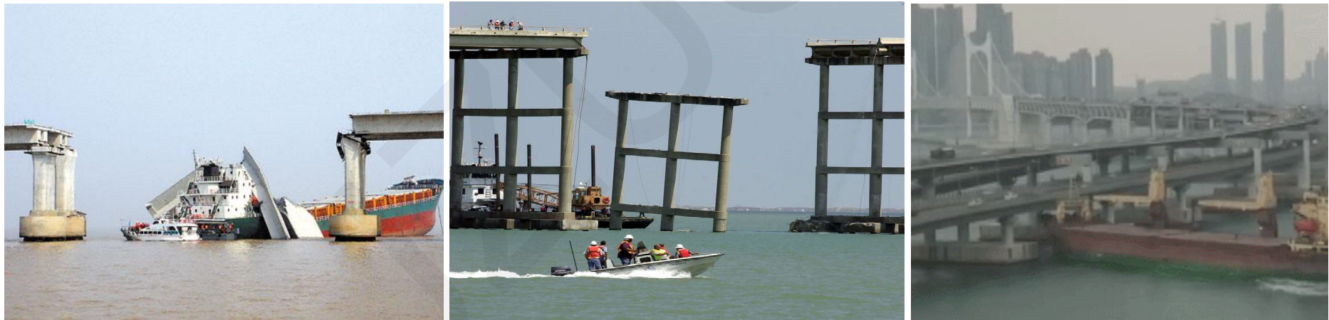
The accident of ship-bridge collisions
