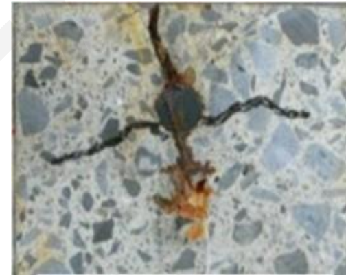
Scenario of a Single Rebar
