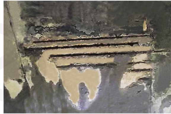
(a) Spalling
