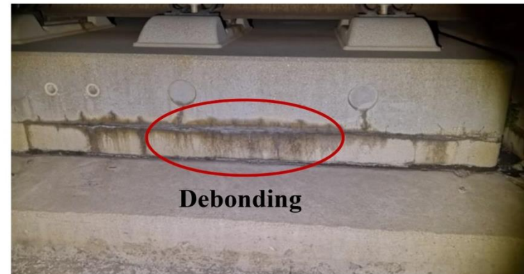
Interlayer debonding between the track slab and SCC
