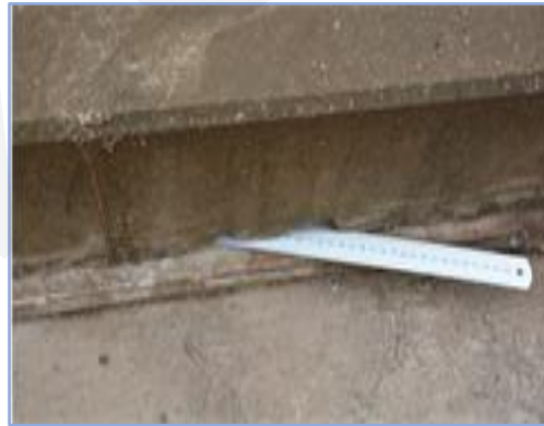
Interlayer debonding between the track slab and SCC
