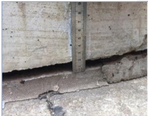
Interlayer debonding between the track slab and SCC
