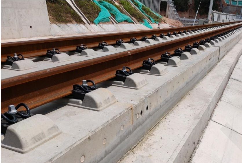
Structural composition of CRTS III prefabricated slab track
