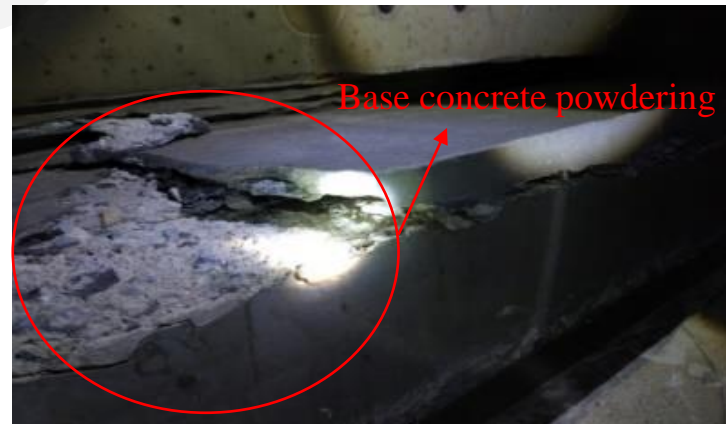
Low temperature causes damage to ballastless track
