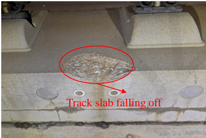
Low temperature causes damage to ballastless track
