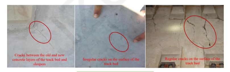
Concrete track bed cracks
