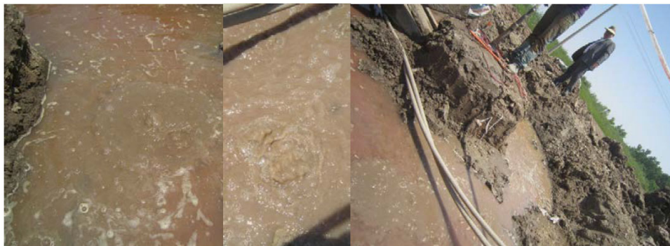
Fig. 8 Slurry breakout phenomenon of the in-situ slurry fracturing tests
