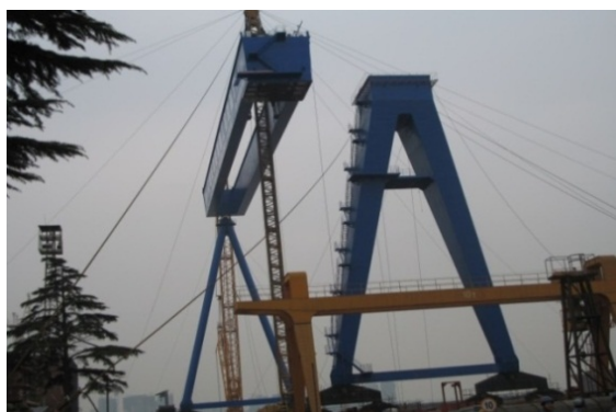
Fig. 11 Gantry crane structure
