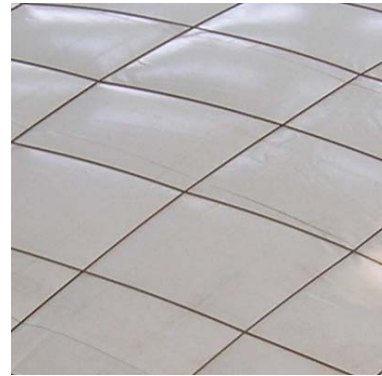
Fig. 6 Contact of cable and membrane
