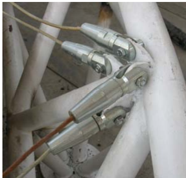
Fig. 5 Anchor device at cable end
