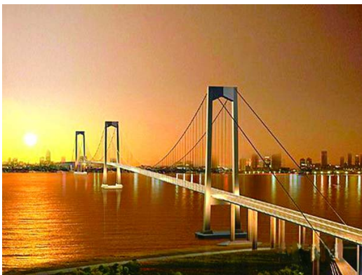
Fig. 2 The Taizhou Triple-tower Suspension Bridge
