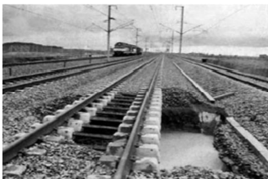
Fig. 1 Unsupported track section (Brabie, 2005)
