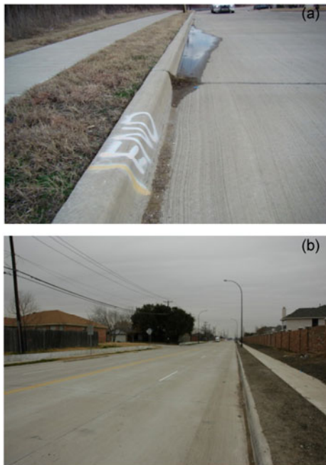
Fig. 4 Photos of control site (ponding) (a) and test site (no ponding) (b) of Southeast Parkway after years of service
